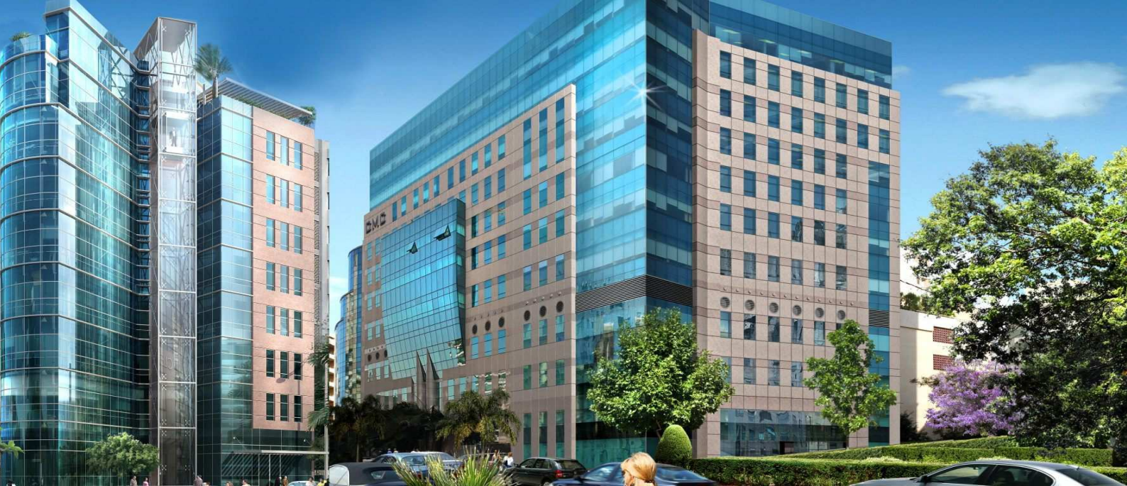
2235 frames, doors and rolling shutters installed at Clemenceau Medical Center Amman are supplied by Fitzpatrick
