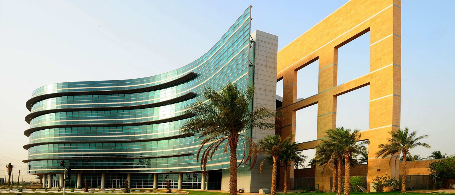
2082 metal frame installed at Kuwait National Petroleum Corporation KNPC are supplied by Fitzpatrick
