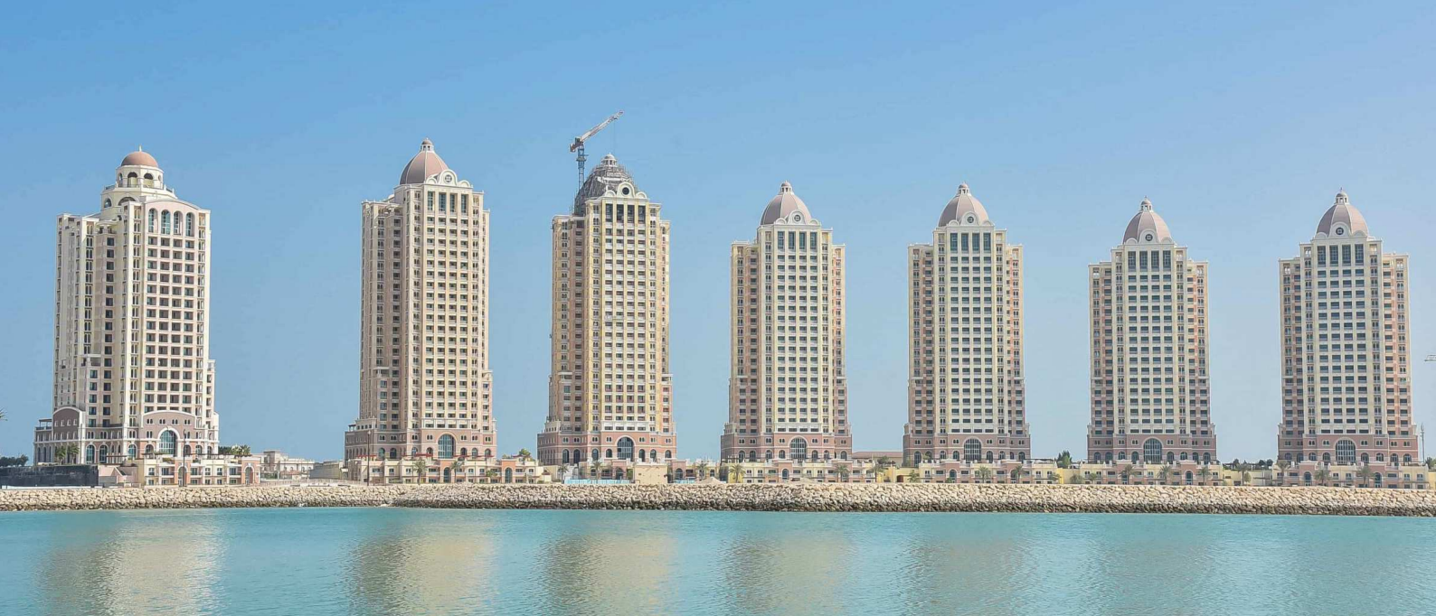
1307 fire rated metal doors installed at Viva Bahria Towers Doha are supplied by Fitzpatrick
