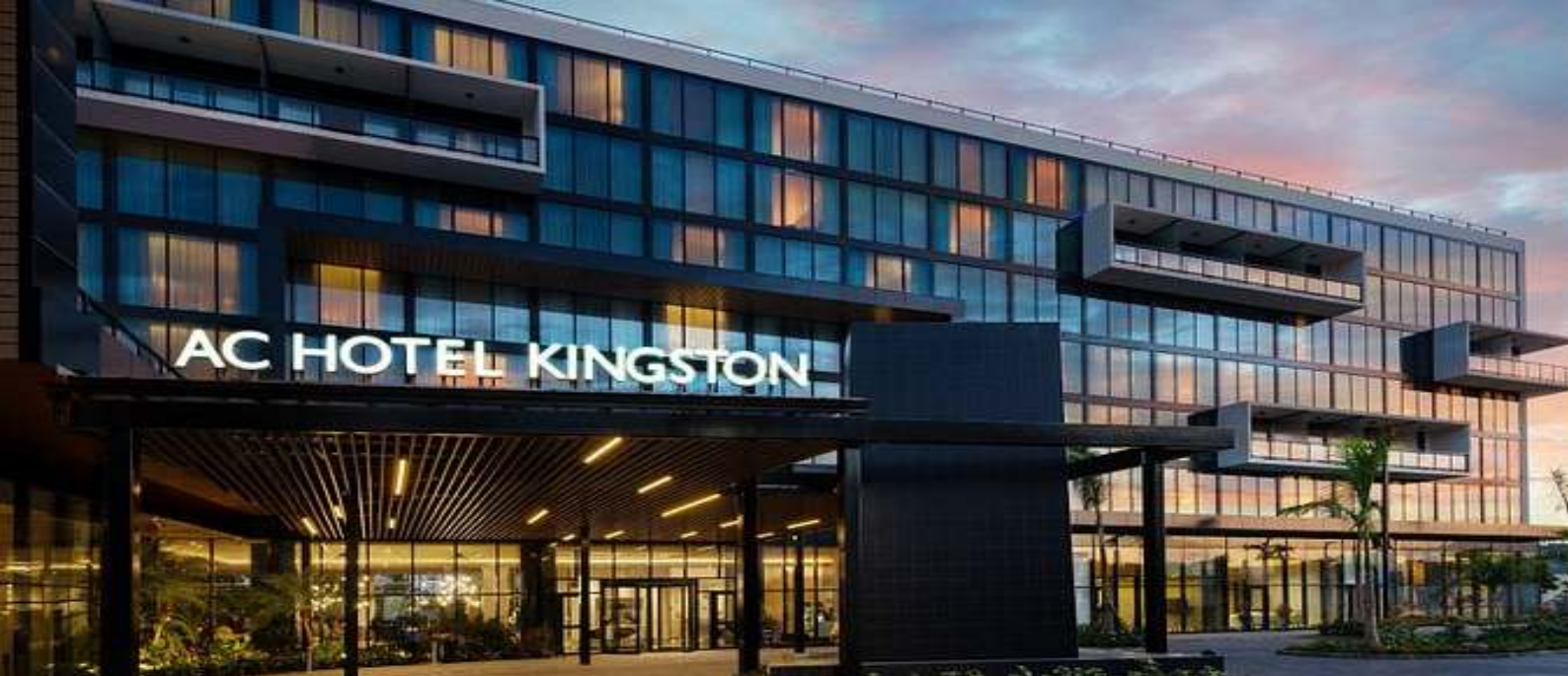
119 frames installed at AC Hotel by Marriott Kingston - Jamaica are supplied by Fitzpatrick
