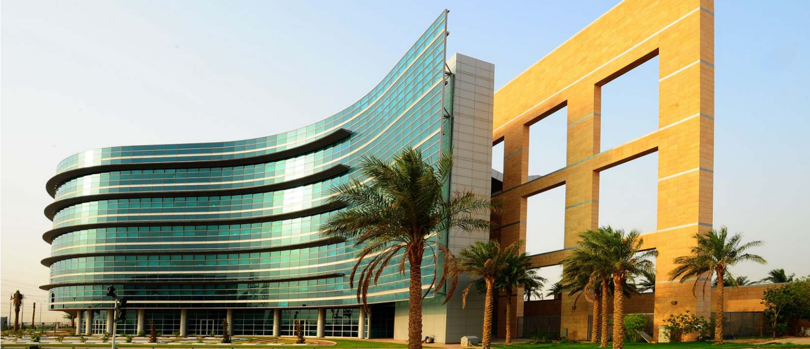
2082 metal frame installed at Kuwait National Petroleum Corporation KNPC are supplied by Fitzpatrick
