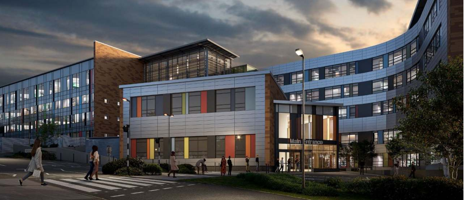
2660 fire rated doors installed at Queen Alexandra Hospital - UK are supplied by Fitzpatrick
