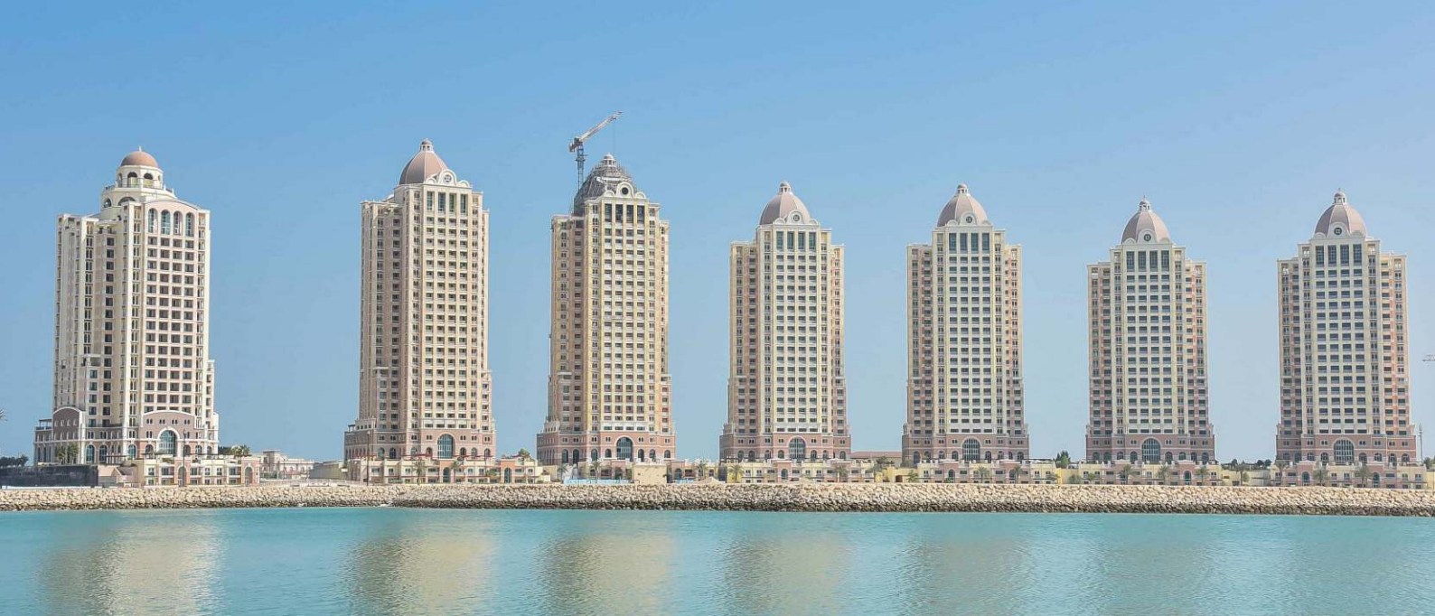
1307 fire rated metal doors installed at Viva Bahria Towers Doha are supplied by Fitzpatrick
