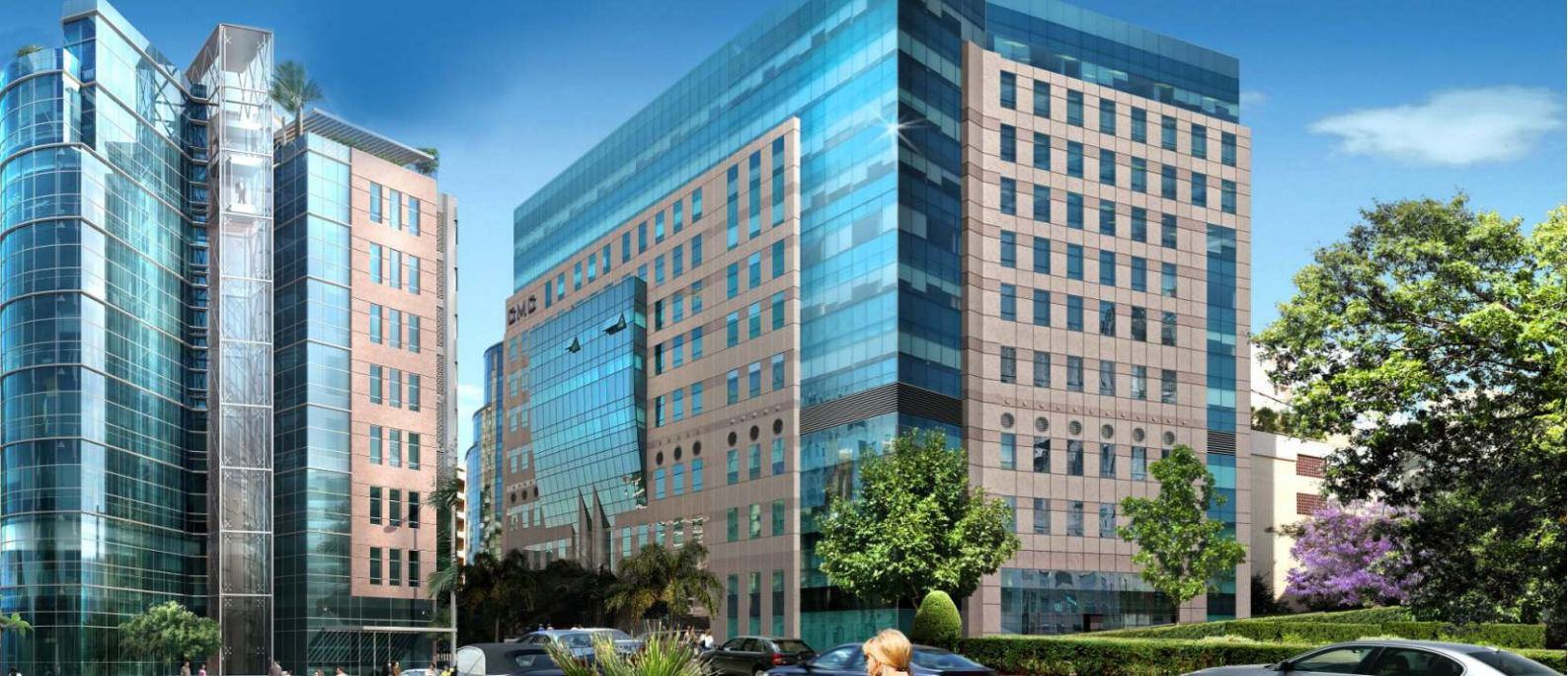
2235 frames, doors and rolling shutters installed at Clemenceau Medical Center Amman are supplied by Fitzpatrick
