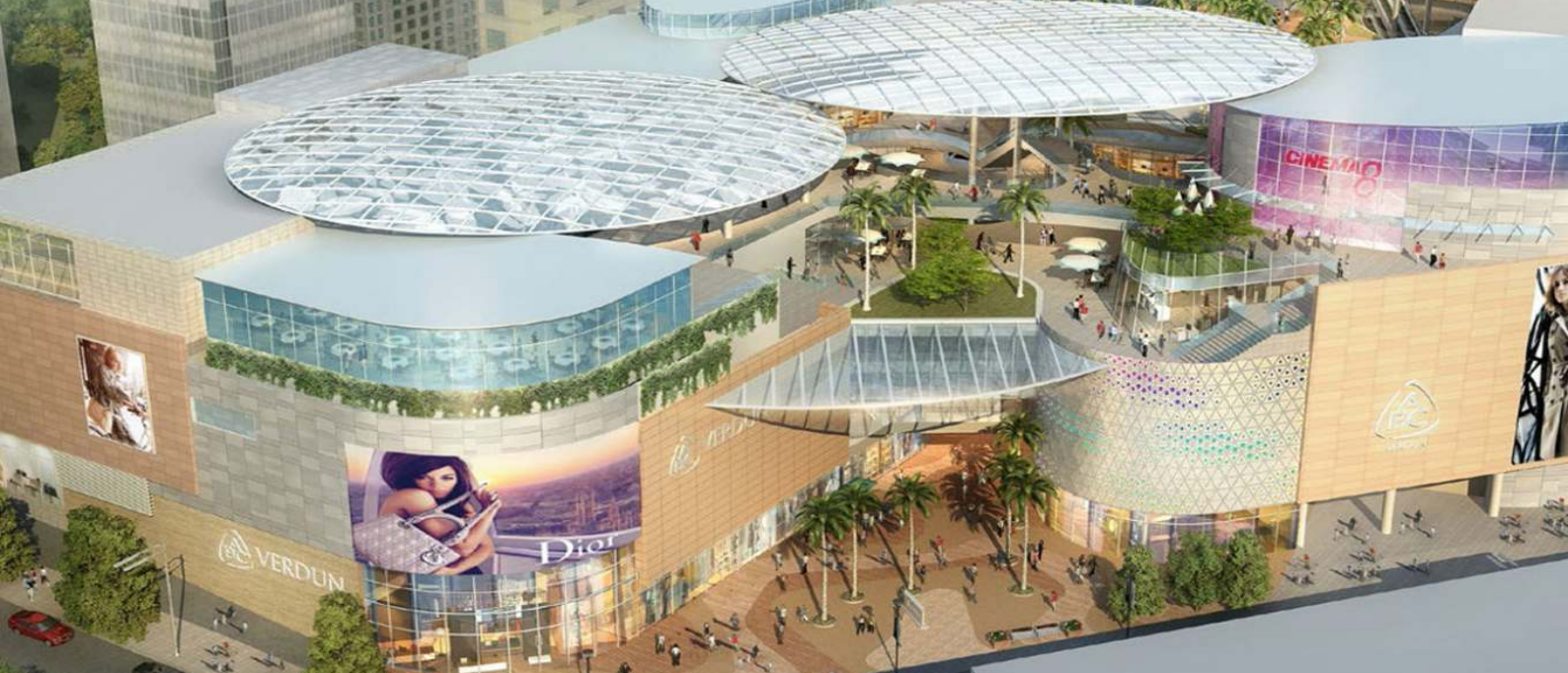
1250 fire rated & main entrance doors installed at ABC Verdun Mall were supplied by Fitzpatrick
